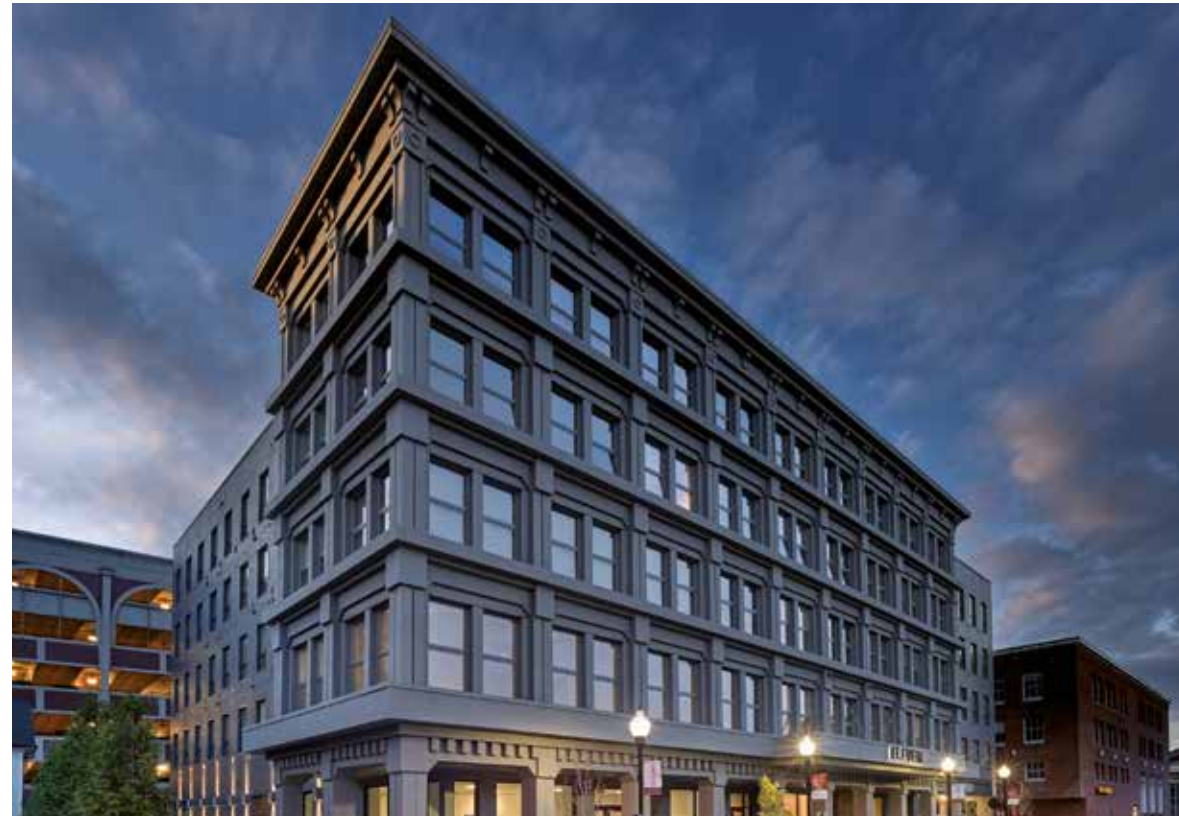
Collective housing, Morrystown (USA) Architect: Marchetto Higgins Stieve Architecture
