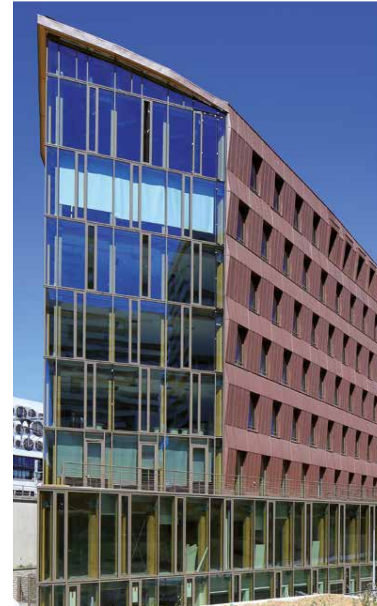
Offices, Paris (France) Architect: Anne Carcelen
